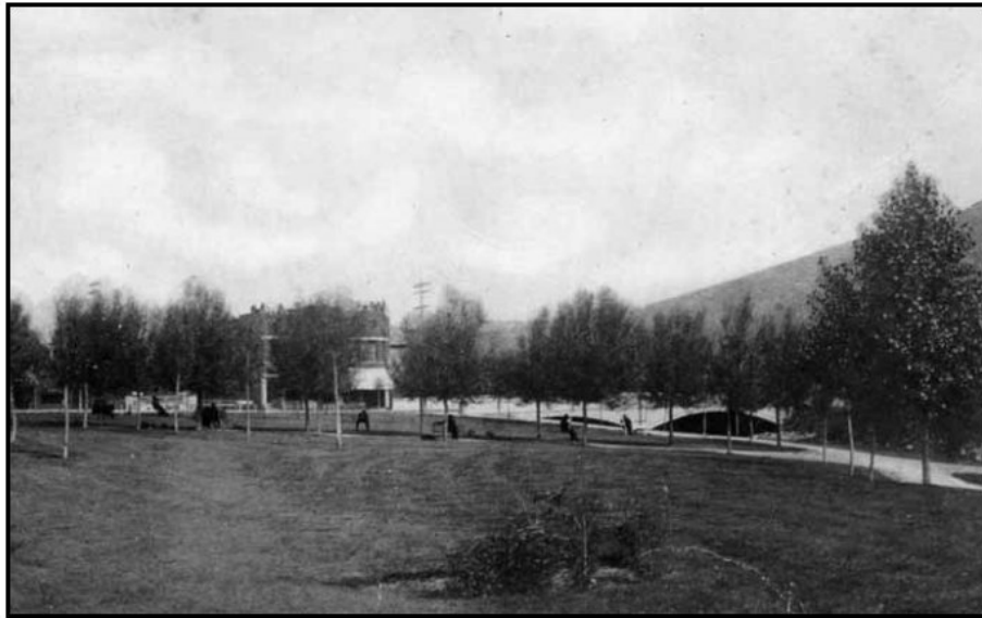
Figure 8. Riverside Park, the Bon Ton/Manhattan Hotel (228 N. F Street), and the current concrete arch bridge over the Arkansas River are shown in this undated postcard view. SOURCE: “Riverside Park, Salida, Colorado,” historic postcard, number 342, Thayer Publishing Co., Denver, Colorado, in the authors’ collection.
