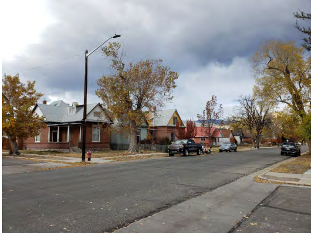
Photo 73: 700 Block F Street looking north
