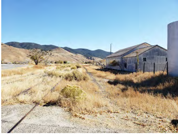
Photo 47: D&RG tracks originally constructed in 1880 between Texas Creek and Leadville with Salida as the major junction. Photo taken at County Road 175 crossing north of town.
