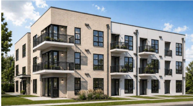
10th and Wolff, Denver. 23 affordable for-sale condominium units.
