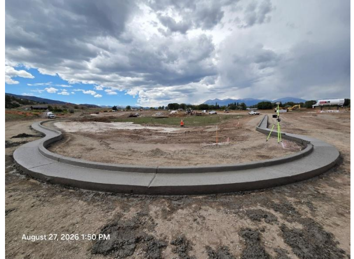
South Ark Neighborhood Curb Installation
