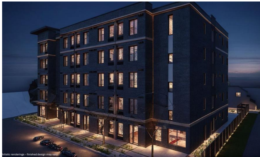
Cherokee Place, Englewood, Colorado. 55 workforce rental units over 2,500 SF of affordable artist live-work space.
