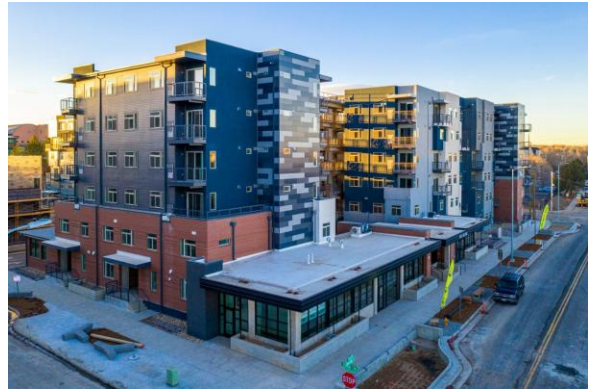
Gateway, Denver. 92 and 95 units across two phases.
