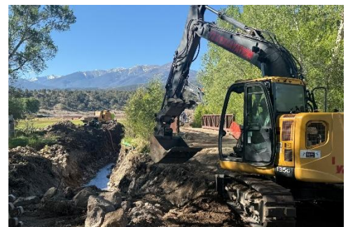
Figure 1- Water Main River Crossing at Pedestrian Bridge
