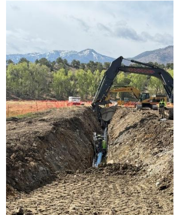
Figure 2-South Ark Neighborhood Water Installation
