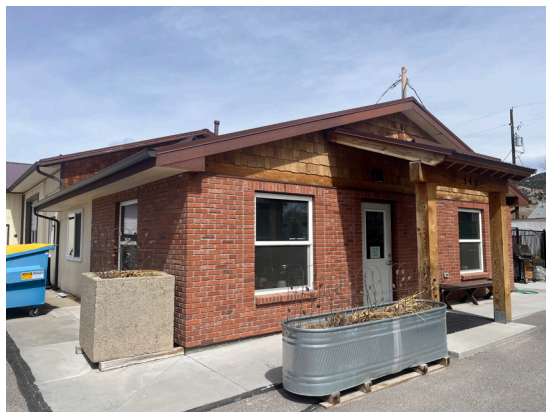
Figure 2-28: Front facade, customer entrance, of the Public Works Facility.
