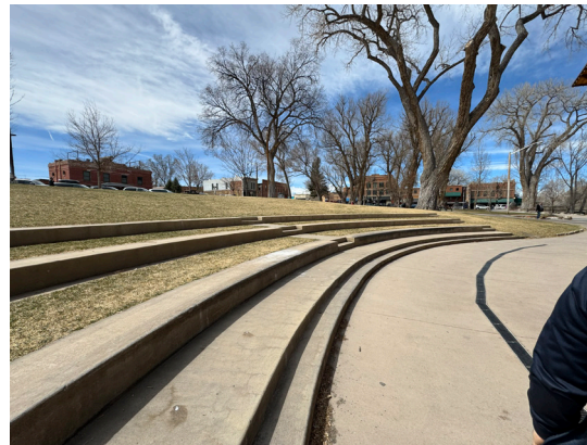
Figure 2-14: Top: Outdoor stadium with stepped hillside seating. Bottom: Tiered hillside seating looking southwest from the amphitheater stage.
