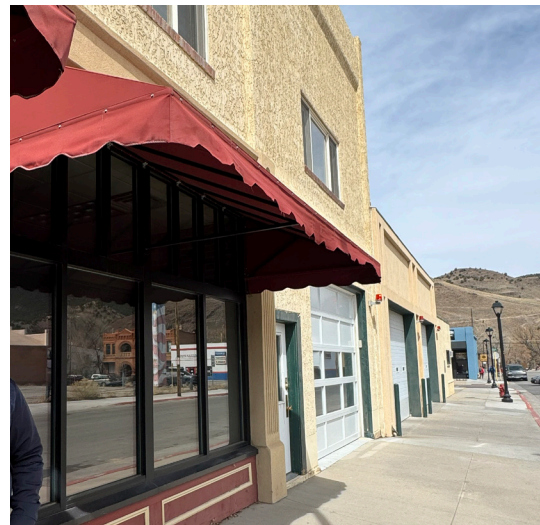
Figure 2-4: Top: East 1st Street Old Fire Station northeast facade. Partially vacated in 2024. South Arkansas Fires Protection District utilizes a portion of the facility for equipment storage. Bottom: Old Fire Station east facade. A portion of the building has two-story office space which is currently vacated.
