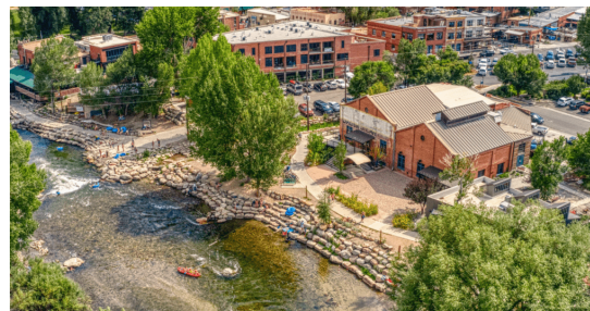
Figure 2-20: The two photos above show the location of Boat Ramp Park in the context of the surrounding buildings and river.
