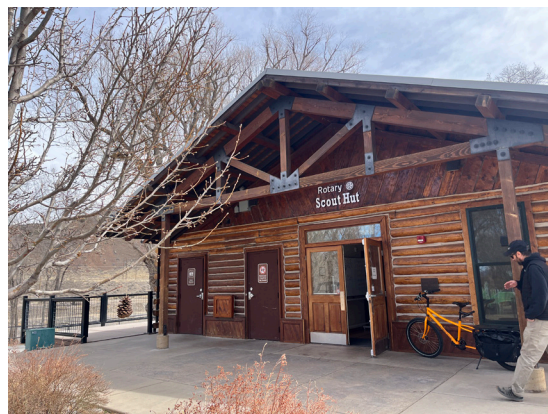
Figure 2-33: Scout Hut main entry and front facade.
