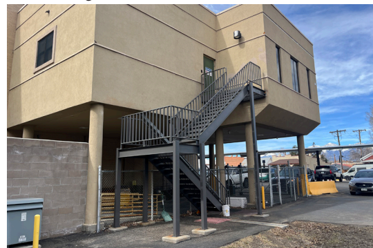
Figure 2-9: Exterior second floor entry to the Police Department. The police utilize this as their main staff and personnel entrance.
