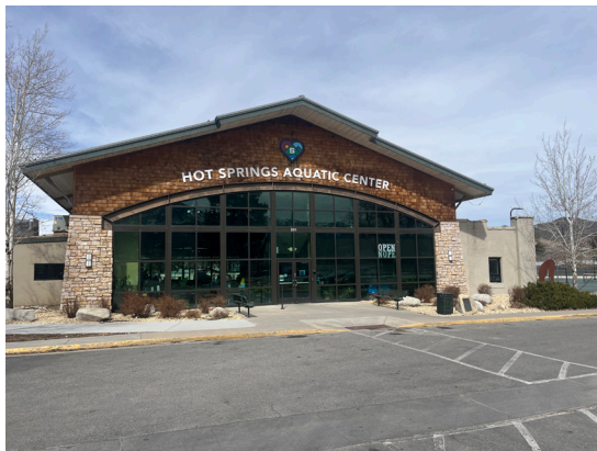
Figure 2-16: Front facade of the Hot Springs Aquatic Center located in Centennial Park.
