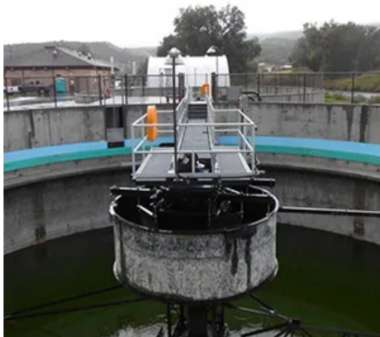
Figure 2-31: Salida Wastewater Plant.
