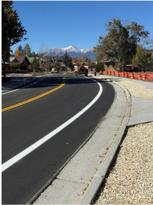
Figure 1 - Oak Street Reconstruction Completion
