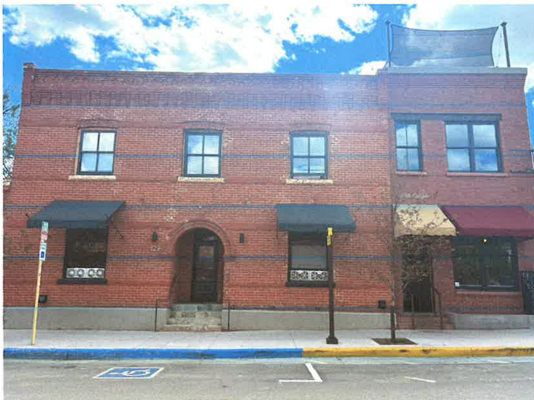
Photo (6): Sackett Ave view of renovated non-contributing building on left and new building on right. Proposed enclosure in upper right where shade sails are shown
