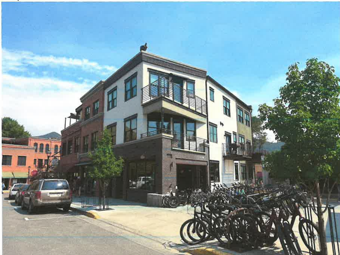
Photo (4): This photo shows the new building that we built on the vacant portion of the lot . Again, this photo was taken from the Southwest corner of the lot
