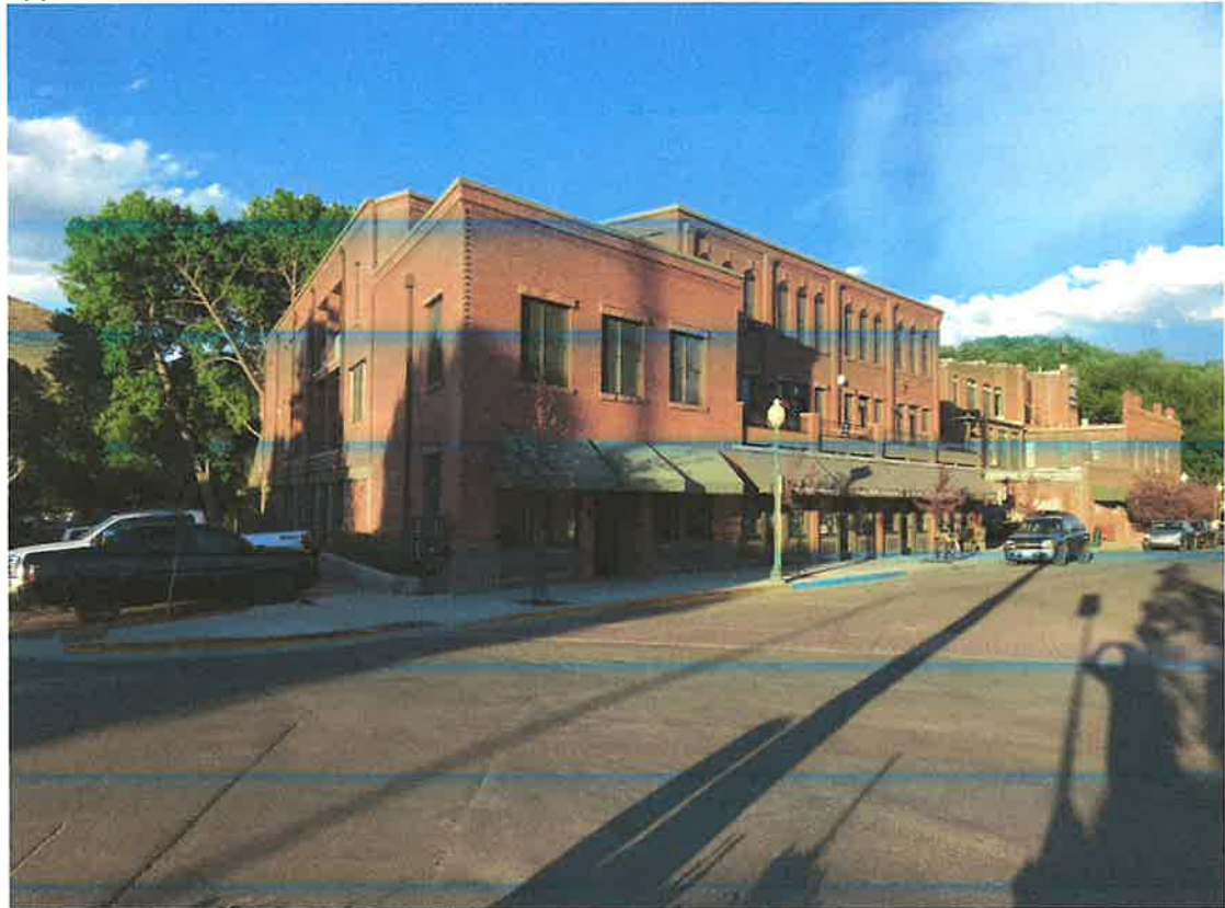
Photo(8): Buildings on north side of W. Sackett Ave, across the street from proposed project.
