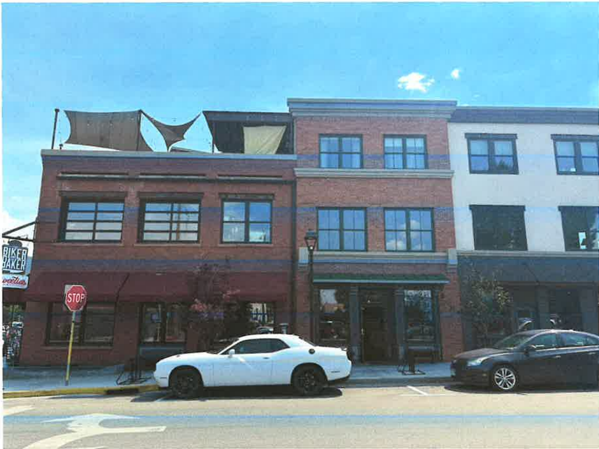
Photo (7); Current 'G' St. view of new building. The proposed enclosure for the rooftop patio is in the upper left where the tiki bar and the shade sails are shown.
