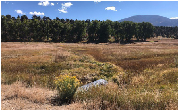
Natural spring and wetlands area and culvert.
